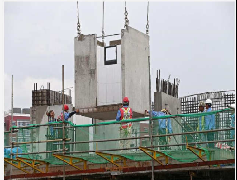
Prefabricated bathrooms units are assembled with finishes in a factory before it is transported to a construction site for installation. PHOTO: LIANHE ZAOBAO
