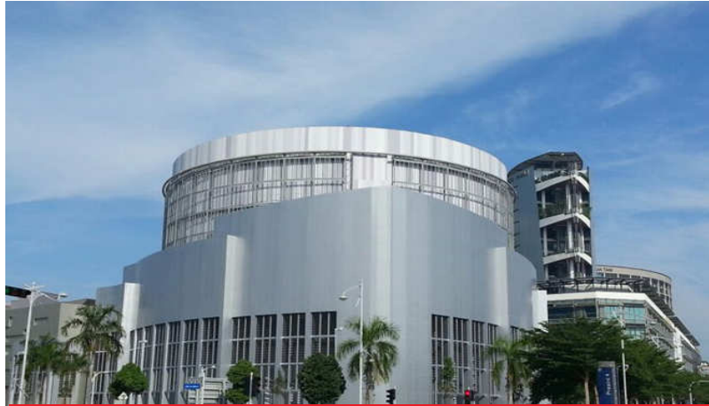
Gas District Cooling Plant
